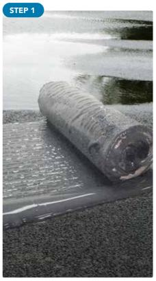
Application of **STARFLEX HYBRID** directly on concrete or sheath, even in the presence of moisture, puddles or rain.
