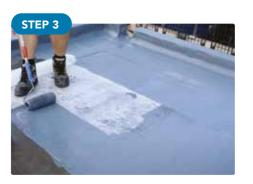
Application of a second layer of **STARFLEX HYBRID** liquid membrane with a consumption of at least 2.5 kg/mq.
