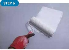
Application of aliphatic polyurethane top coat of the **POLISTAR** line.
