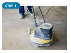
Preparation of the substrate, cleaning and realization of the perimeter flaps.
