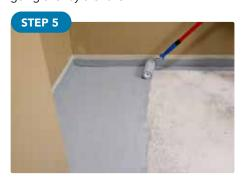
Application of a last coat of **STARFLEX H-ZERO** liquid membrane > 0.6 kg/sqm
