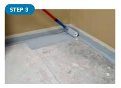
Application of a first coat of **STARFLEX H-ZERO** liquid membrane > 0.7 kg/sqm and application of STARTEX reinforcement, going over by the roller.
