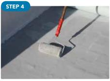
Application of a second coat of **STARFLEX H-ZERO** liquid membrane > 0.7 kg/sqm.
