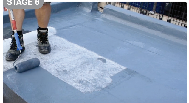
Application of a second coat of STARFLEX liquid membrane.
