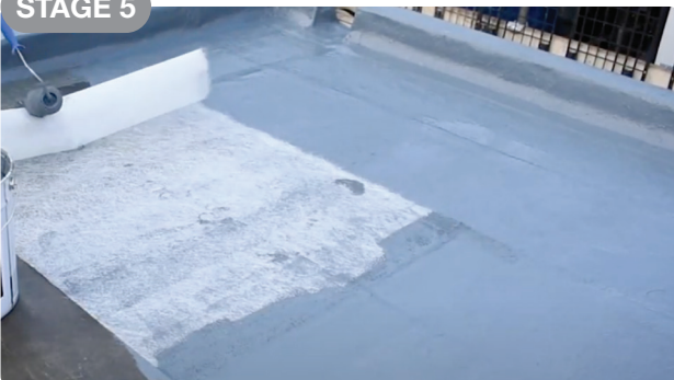
Placement of STARTEX fabric.
