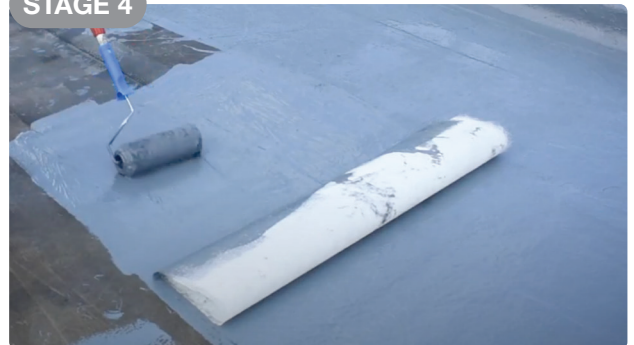
First coat application of STARFLEX liquid membrane.
