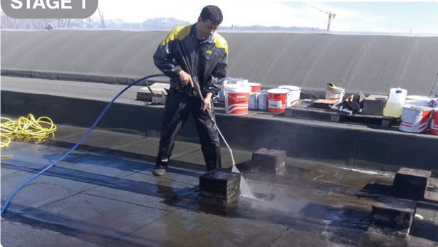
Cleaning of the laying surface and arrangement of the existing one.
