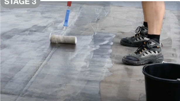
Application of specific primer for the existing laying surface.
